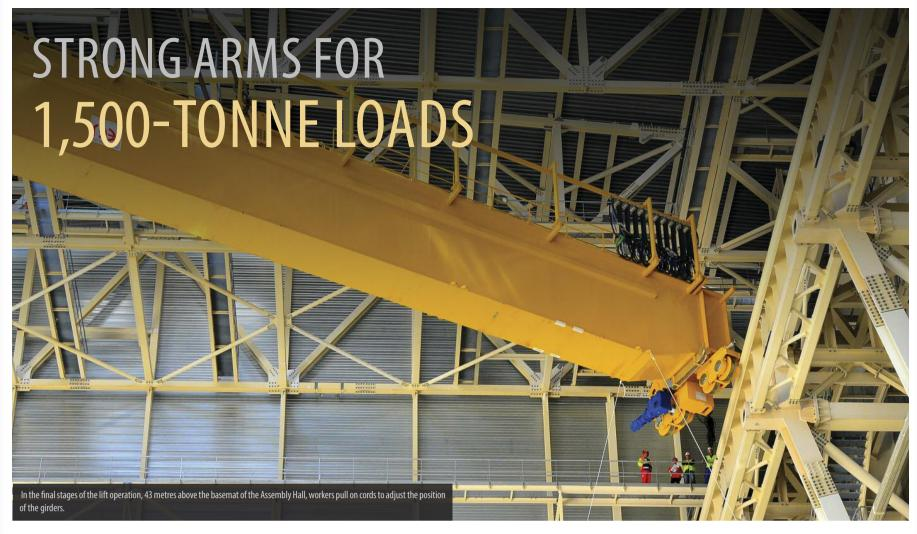
1,500 tonnes – or the equivalent of four Boeing 747s fully loaded with passengers and fuel. That's what the recently installed Assembly Building bridge cranes will be capable of handling when operated together.
